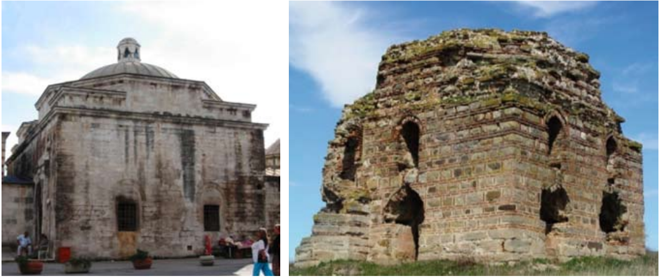
Figure 13. Accumulating black crusts at the north façade of Hızırbey Külliye from Kırklareli (left) and Gazi Turhan Bey Külliye Uzunköprü province in Edirne.
